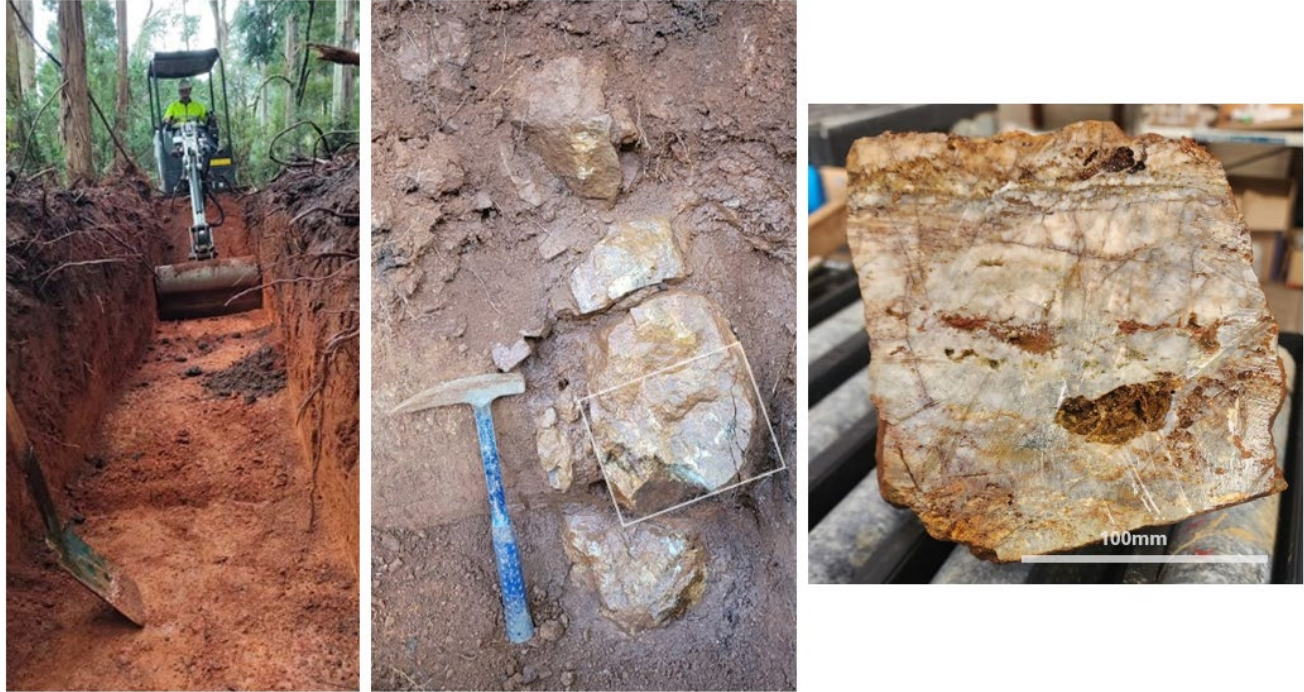
Figure 4 - Left: Flynn Gold trench around 1m wide being excavated down to bedrock using a 1.7 tonne excavator. Centre: In-situ vein up to 230mm wide (200mm average) discovered in the historic trench. Right: Cut sample from in-situ vein (white box centre picture), returned 0.2m @ 48.5g/t Au (Sample 75539).
