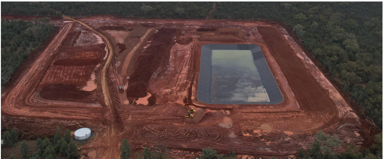
Figure 2: Completed 30ML lined sump dam within the perimeter of the larger 230ML water management dam.
