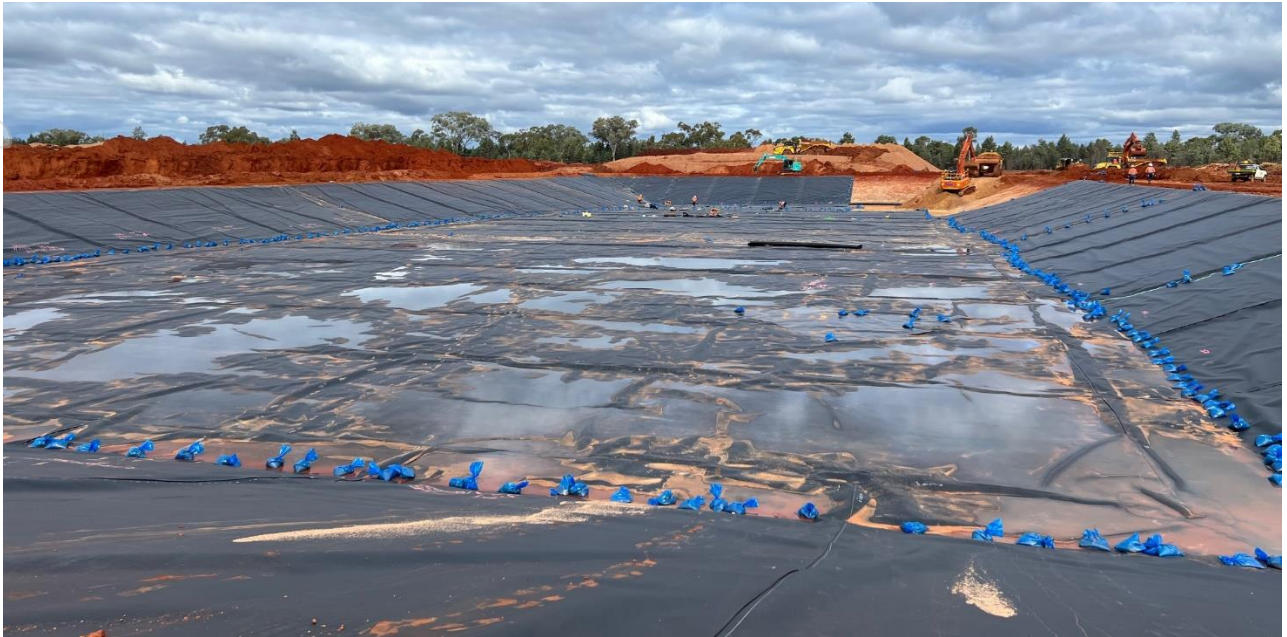
Figure 1: Lining of 30ML sump dam nearing completion.
