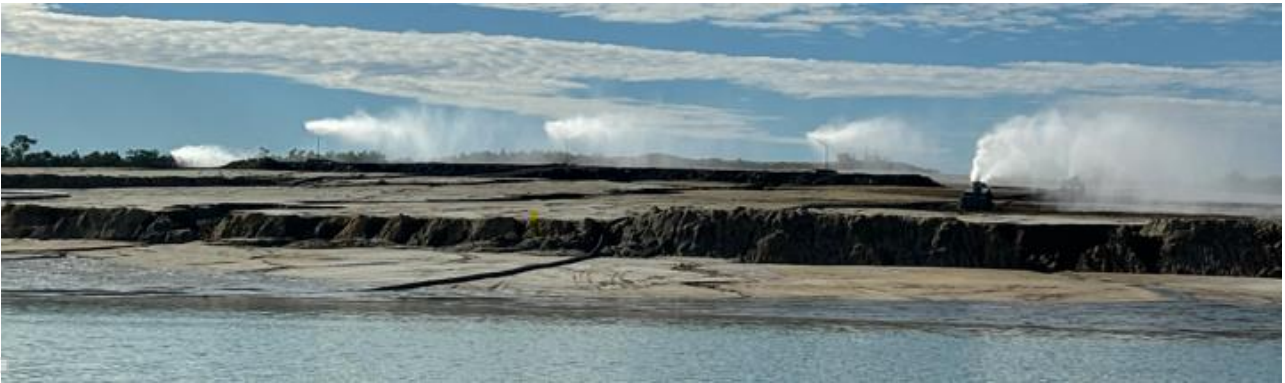
Figure 4: Water cannons and misting evaporators in operation at the Hera TSF.
