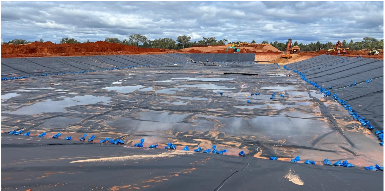
Figure 1: Lining of 30ML sump dam nearing completion.
