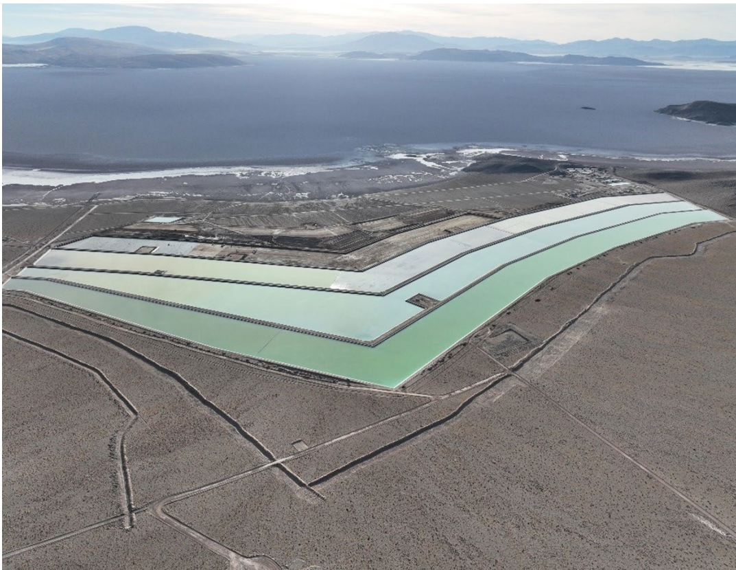
First 3 ponds completed, filled and evaporating
