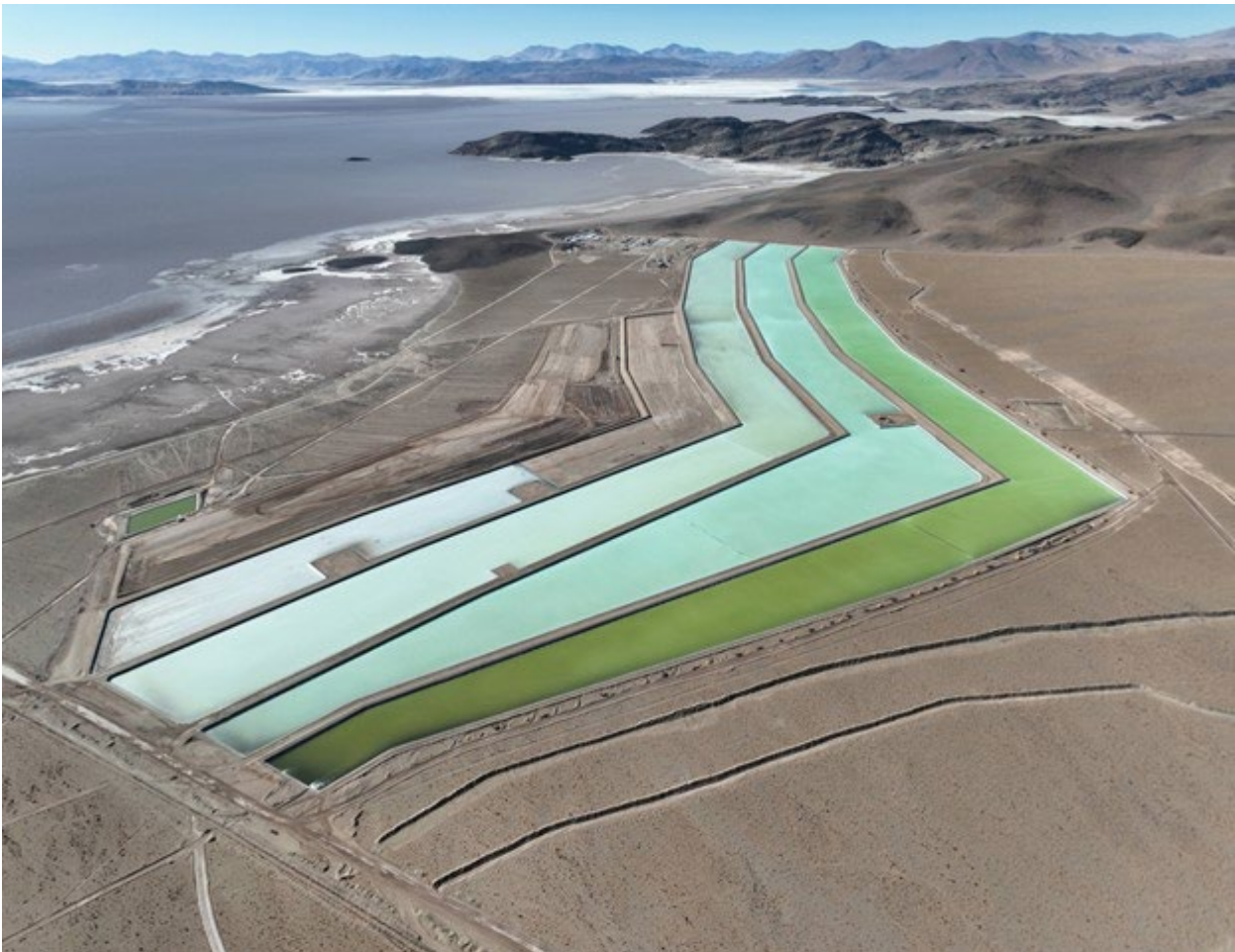
HMW Project looking south
