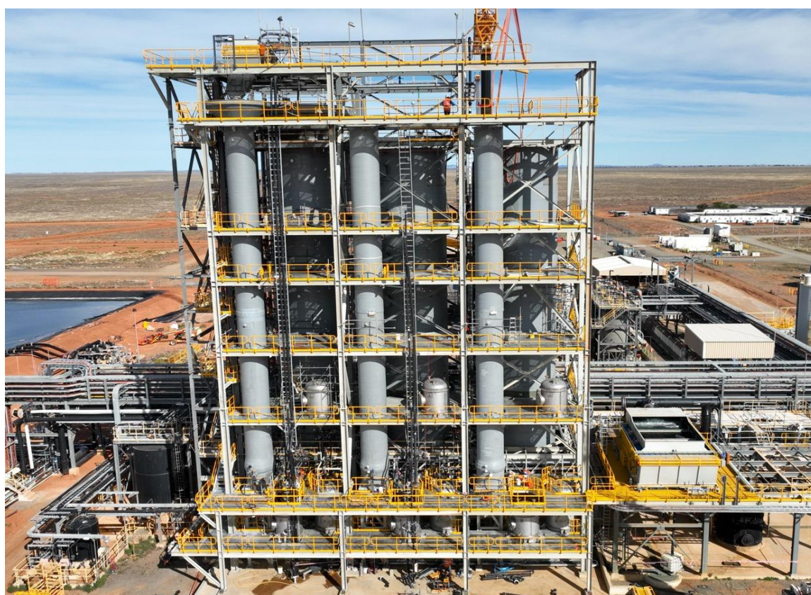
Figure 2: Construction of columns 2 and 3 nearing completion to increase Honeymoon's production profile
