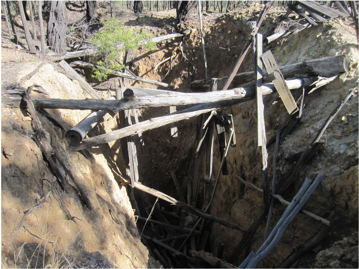
Figure 6 Historic Banshee workings showing unstable shaft requiring protection.
