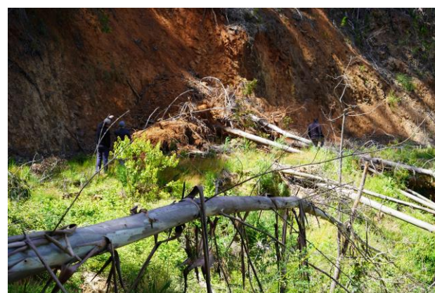
Photo 6 – Exposed clays in Road Cutting
