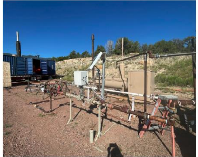
Images 1 & 2: The Pathfinder 1 well (L) and the gas connection point linking to the generator (R)
