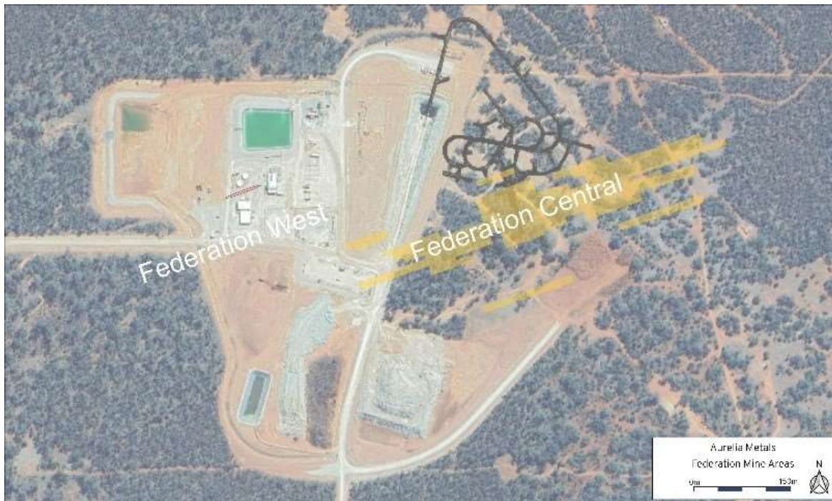
Figures 13: Local location map of the Federation Mine with underground development at mid-May 2024.
