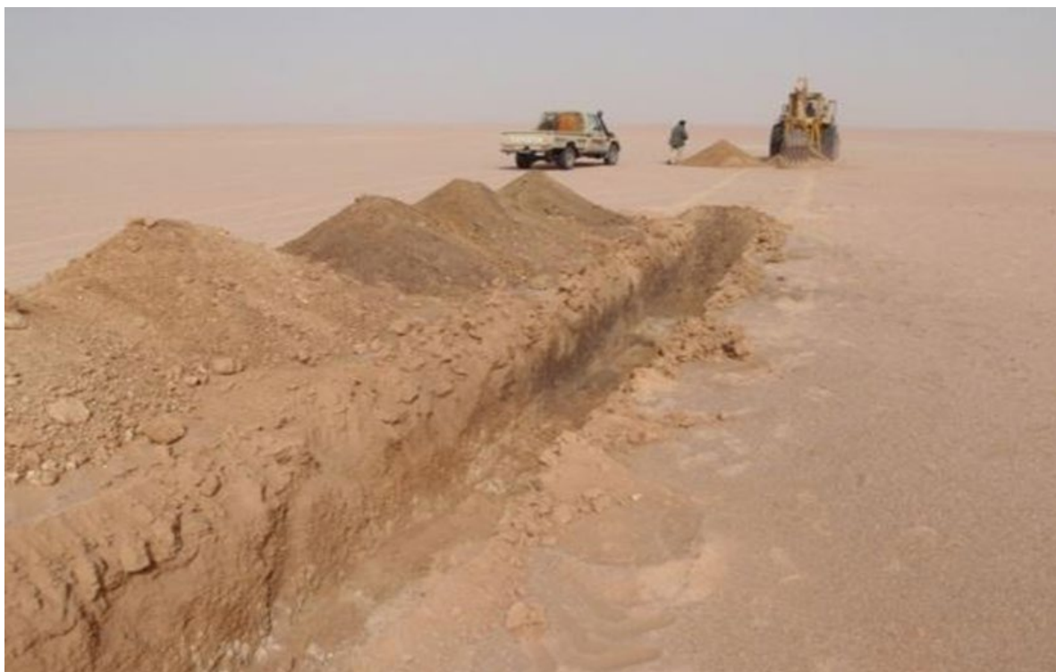
Figure 5: Typical landscape within Tiris project area, trench illustrating soft sandy overburden with gravelly free digging calcrete ore generally less than 6 metres deep.
