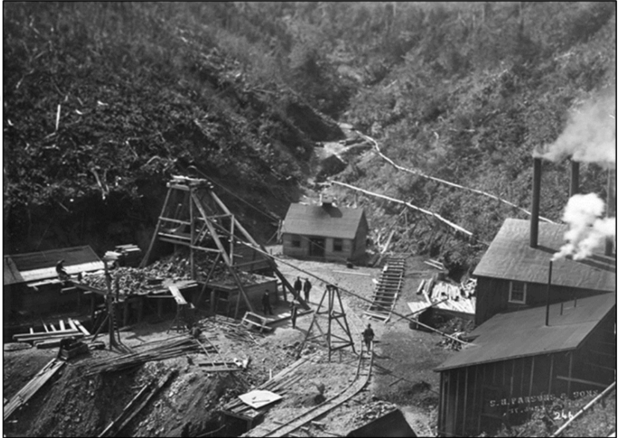
Figure 8: York Harbour “A” Zone Shaft and Mine Buildings (ca. 1899–1913)
