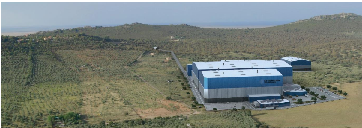
Figure 1: Design Drawing of the San José Lithium Project within the Project area and PESE.
