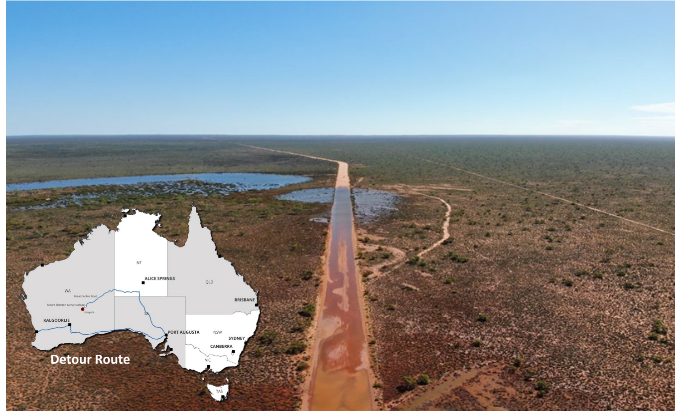
Great Central Road 20 March 2024
