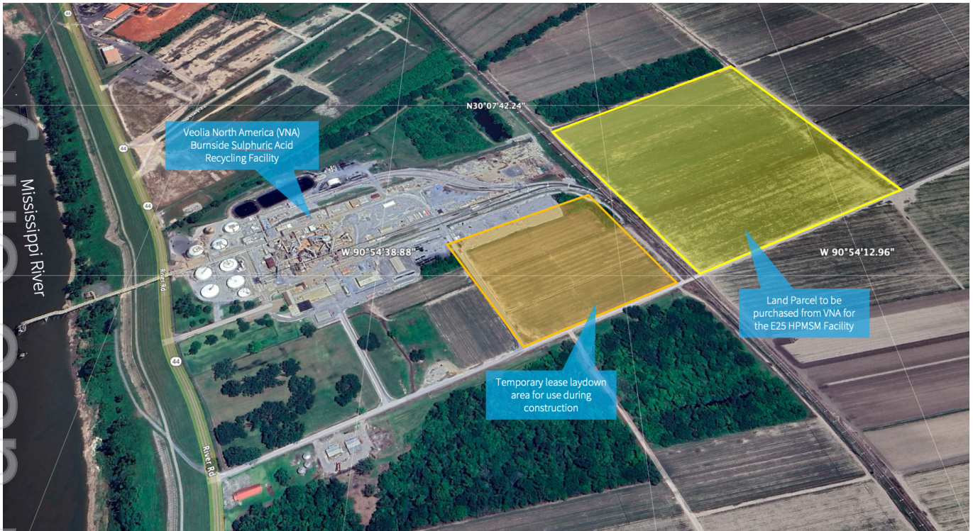
Figure 1. Proposed construction site for the Louisiana HPMSM facility close located with the Veolia North America acid plant.
