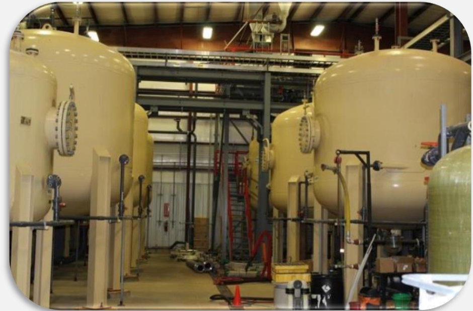
Lance Satellite Plant Ion Exchange System
