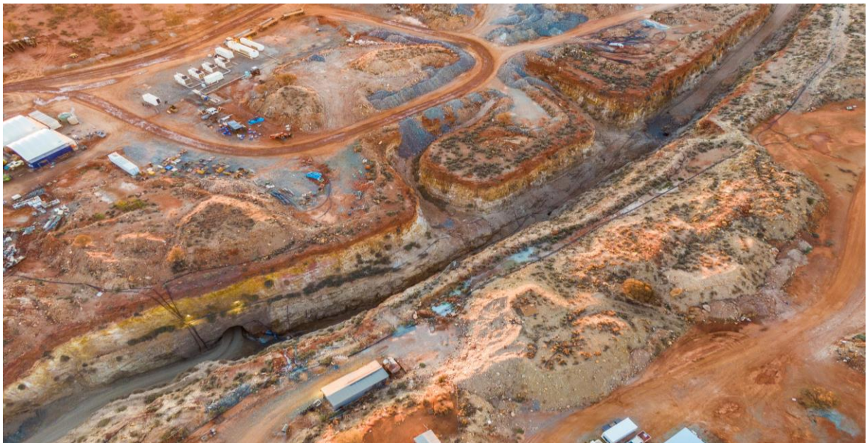
Figure 4 - Second Fortune underground portal
