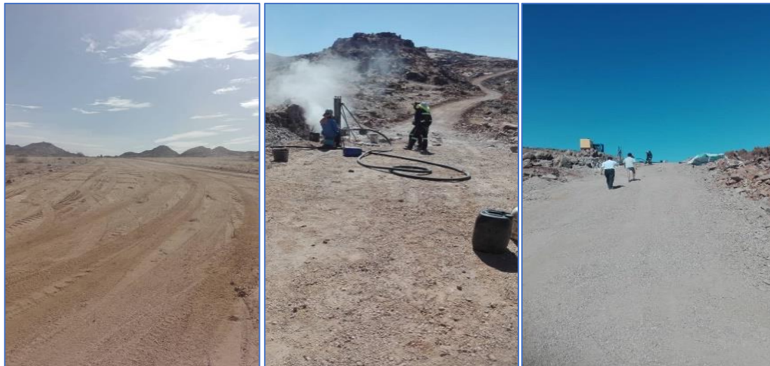
Figure 2 – Completed road between nearest traversable road to Swanson Plant
