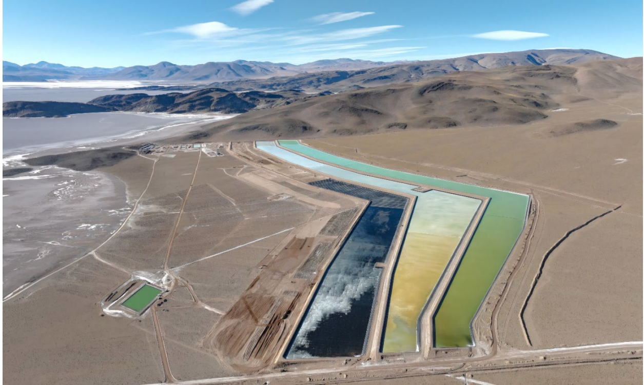
Pond 3 liner installation and Pond 4 earthworks
