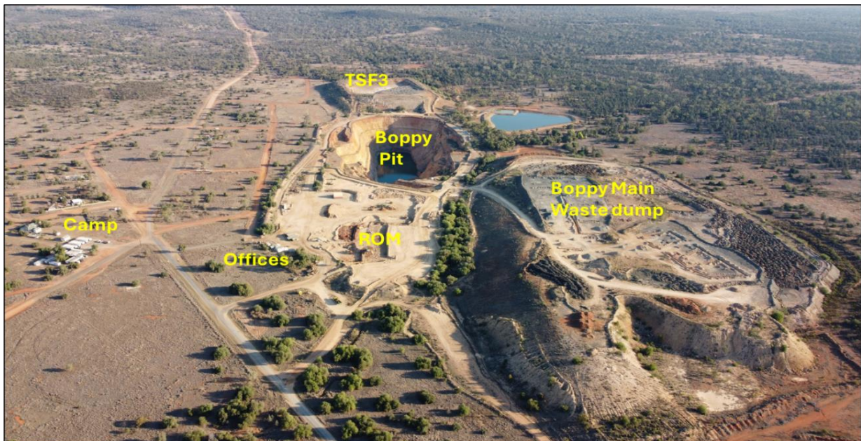
Figure 1: Drone image looking south showing the main components of the Rock Dump and Tailings Resources in relation to the Mt Boppy open pit.
