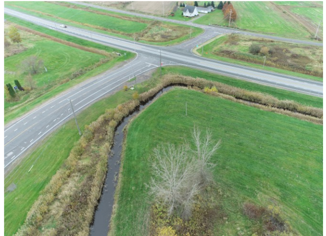
South side of Lot 22 at Bécancour, Québec proximal to highway access
