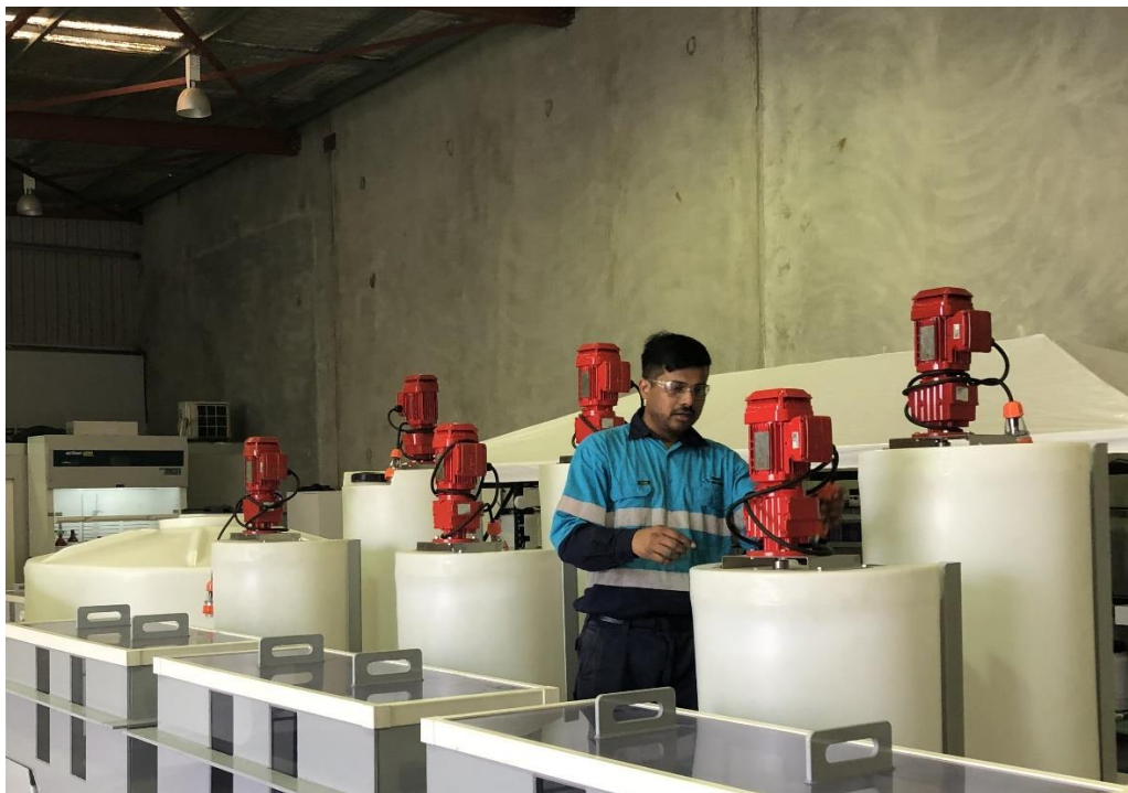
Figure 1 - Process Engineer, Syed Zaidi inspects the delivery of the SX modules.
