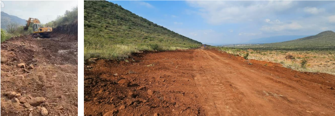
Figure 4: Site preparation for installation of boundary fence
