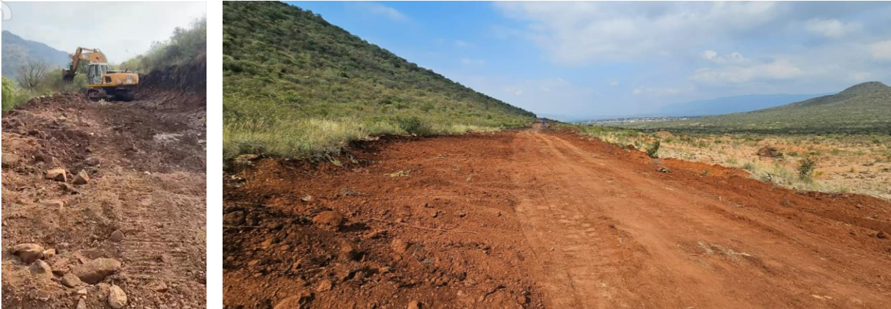
Figure 4: Site preparation for installation of boundary fence
