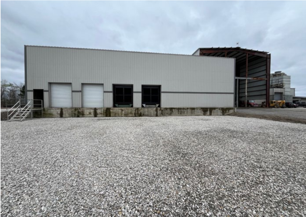
Image 4: New Generation Production Facility (L) and Warehouse Receival/Storage Facilities (R)
