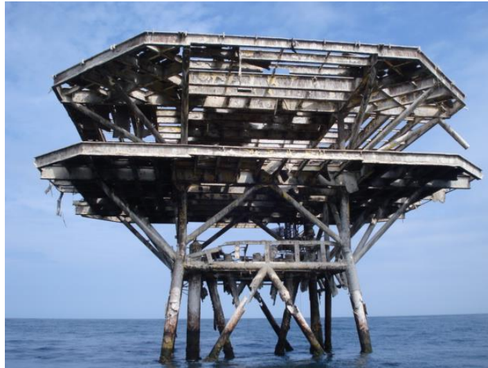
Figure 3 – C-18X well platform
