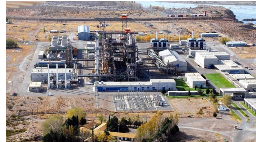
Arroyito Heavy Water facility in Neuquen
