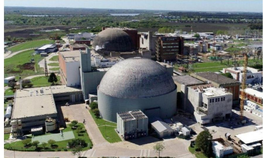
Atucha Nuclear Energy facility in Buenos Aires
