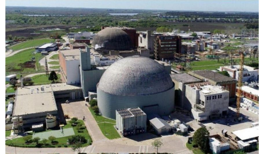
Atucha Nuclear Energy facility in Buenos Aires
