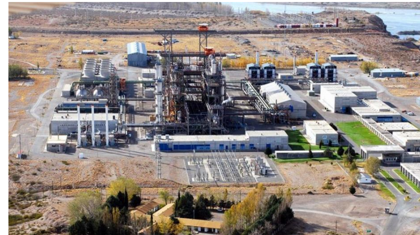
Arroyito Heavy Water facility in Neuquen
