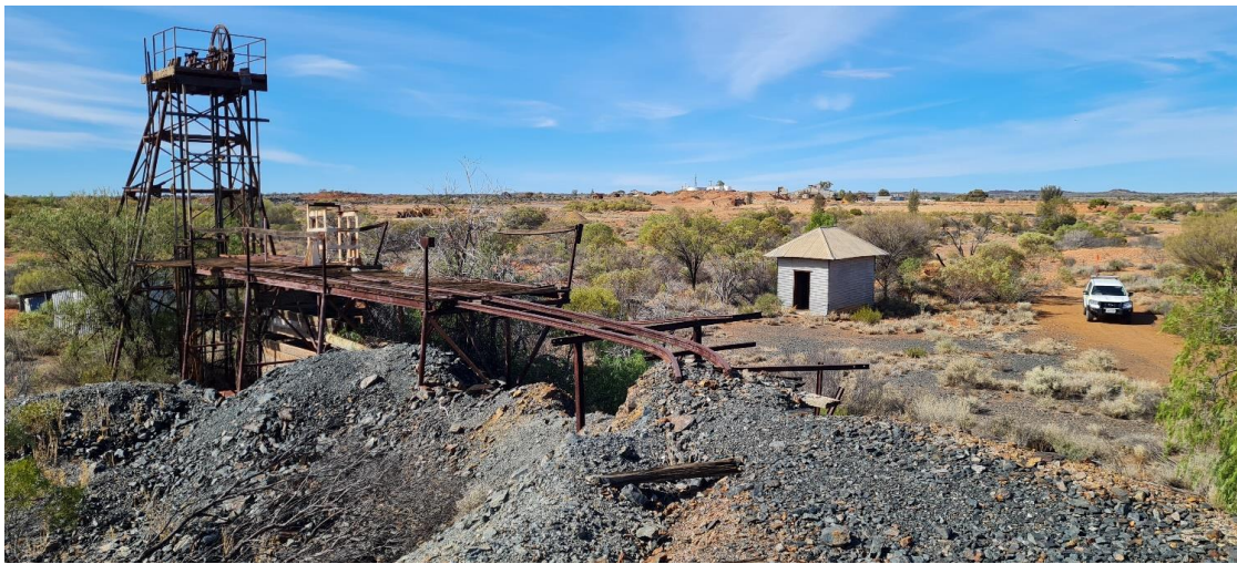
Figure 6 - Aspacia Headframe (looking South East)
