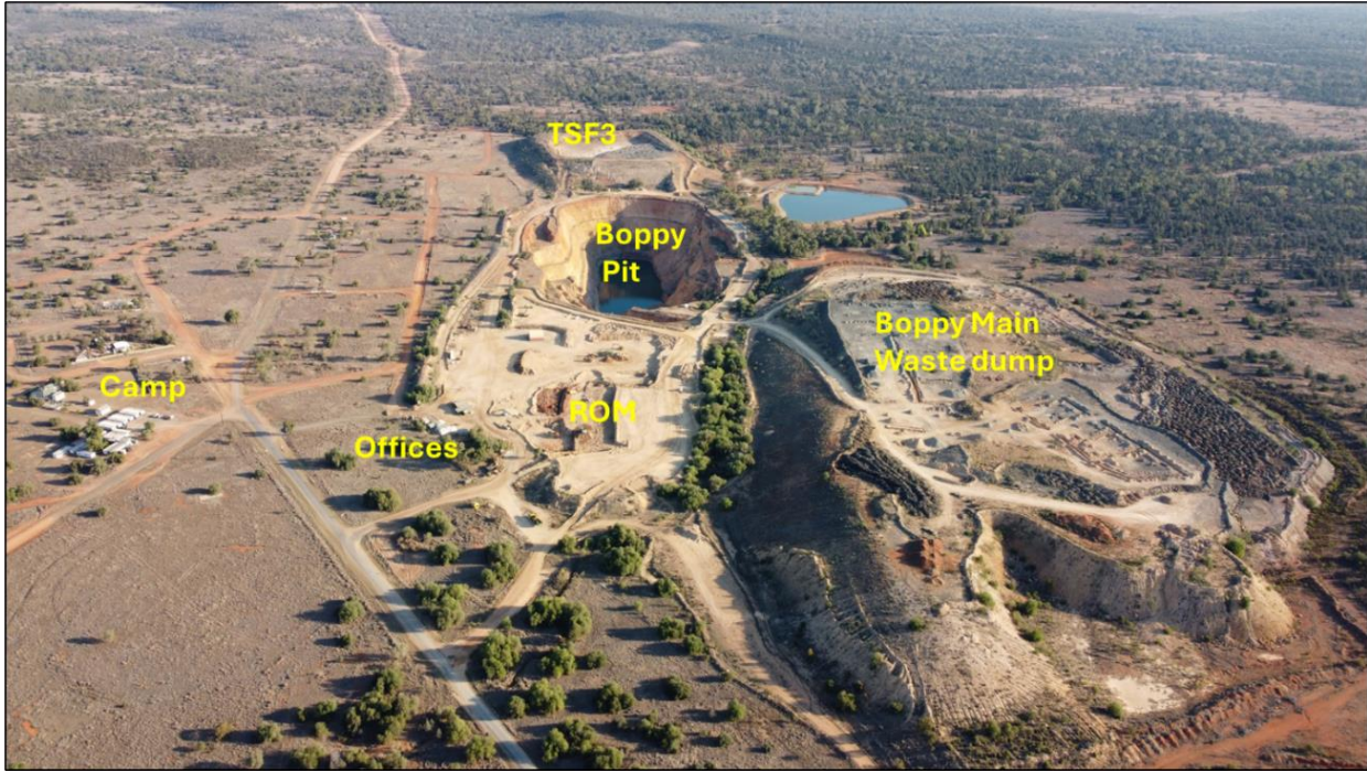
Figure 2: Drone image looking south showing the main components of the Rock Dump and Tailings Resources in relation to the Mt Boppy open pit.
