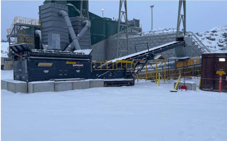
Figure 4 – Refeed System nearing completion
