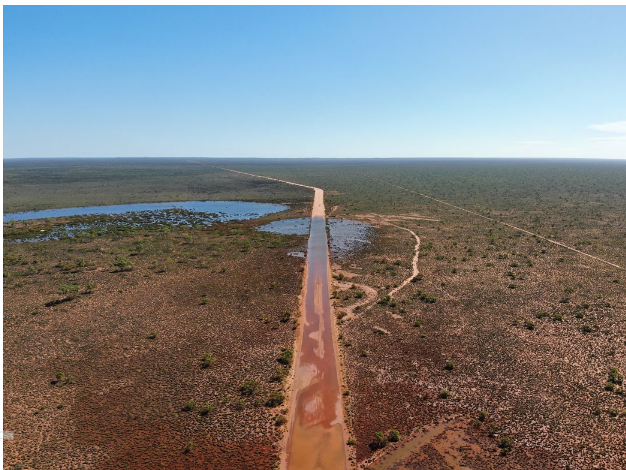
Figure 1: Great Central Road Flooding 20 March 2024
