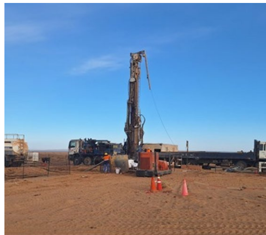
Figure 7: Water Monitoring Bore Drilling
