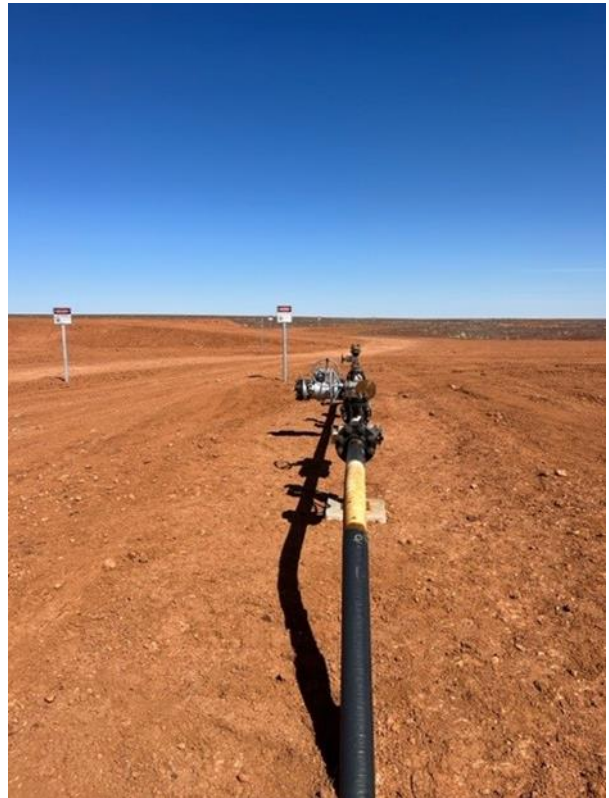
Figures 2 - 4: Yarrow Pipeline Completed (photos courtesy of Santos)
