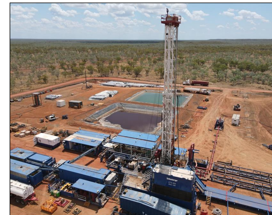
SLB 185 Rig drilling Carpentaria-3H in EP187
