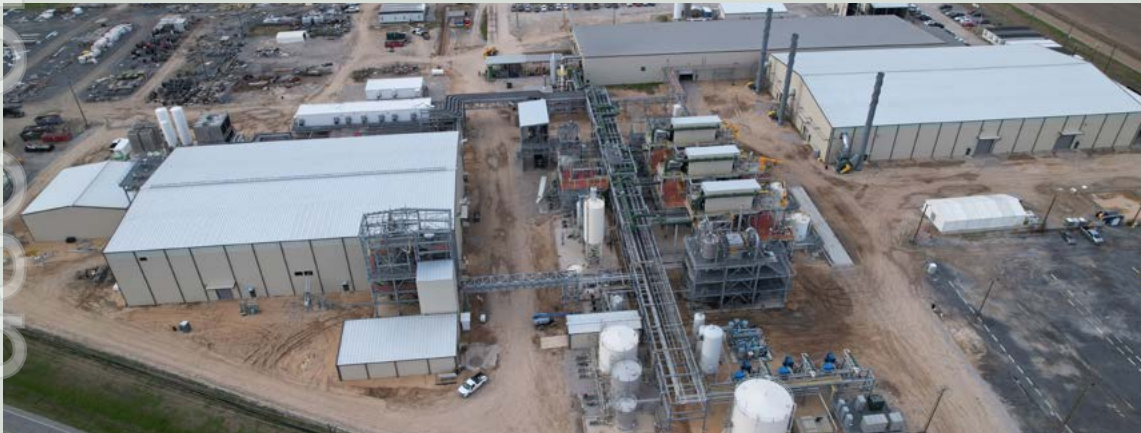
◀ Vidalia AAM facility
