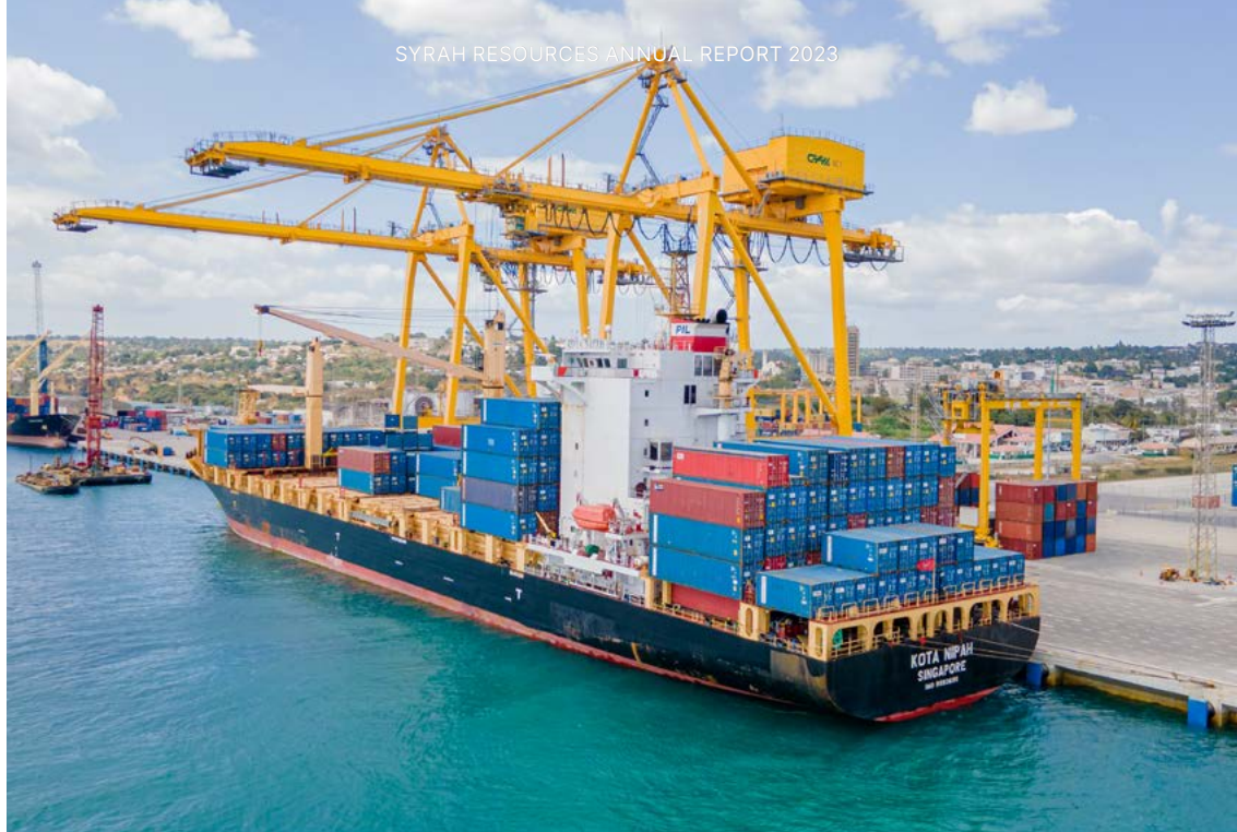
New shore cranes at Nacala port
