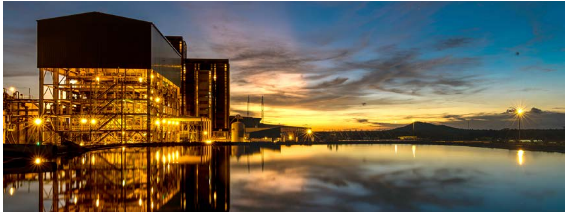
Balama processing plant
