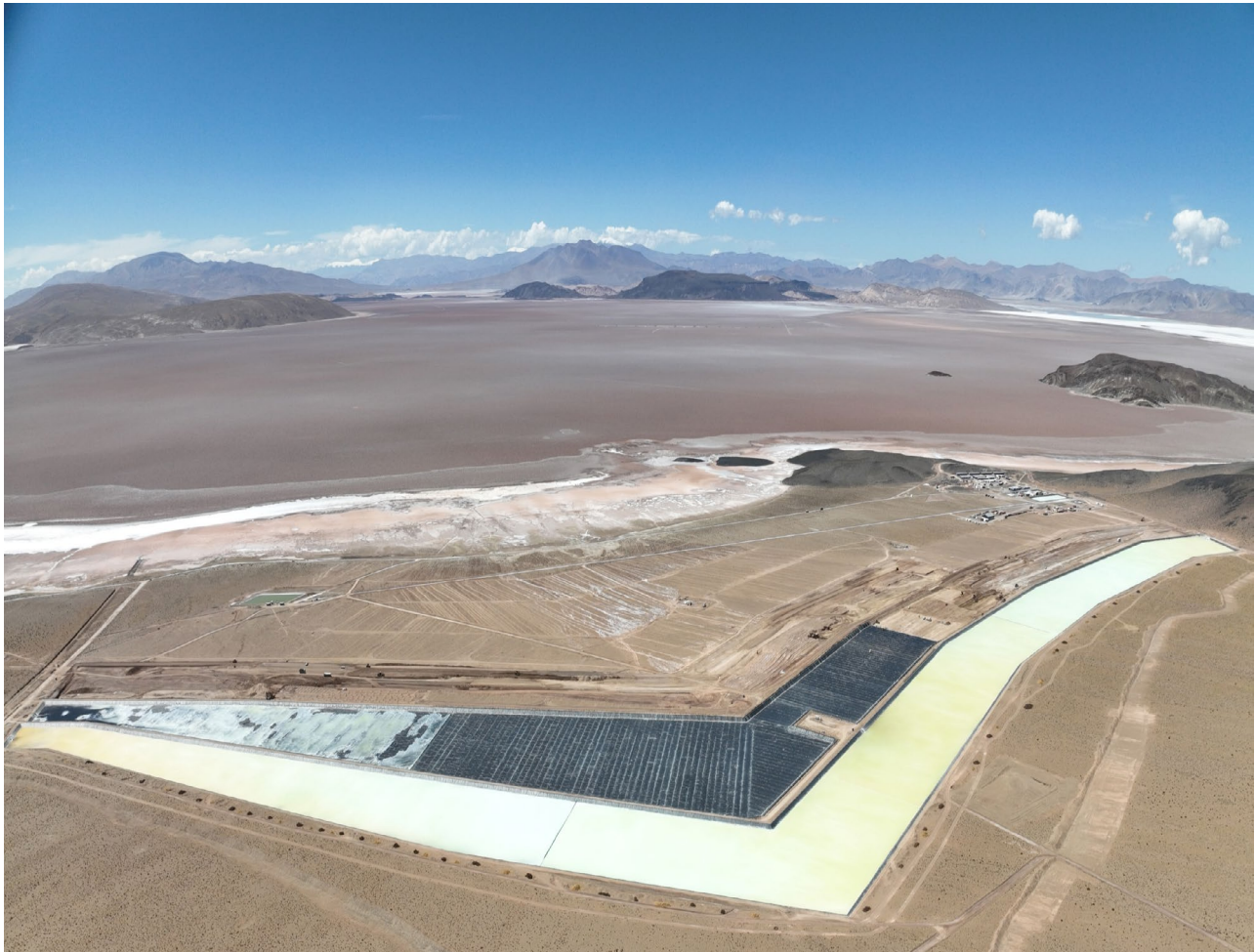
Pond 2 filling has commenced
