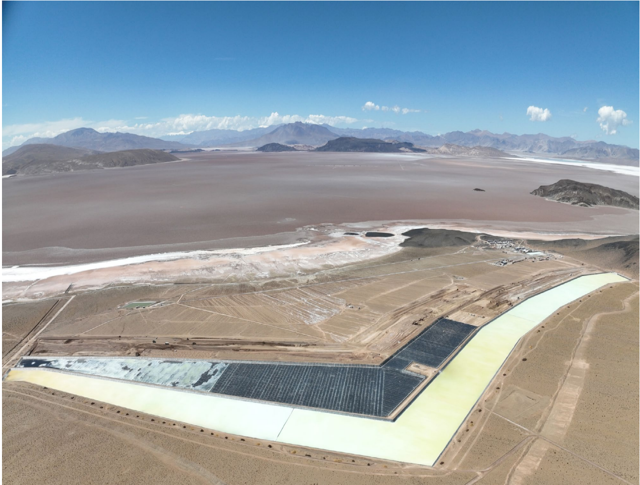
Pond 2 filling has commenced
