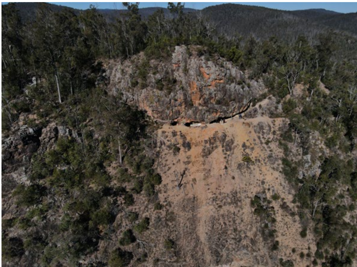
Figure 3: Aerial View of the Cliff Workings and Red Rock Mine (ML) from the exploration licence
