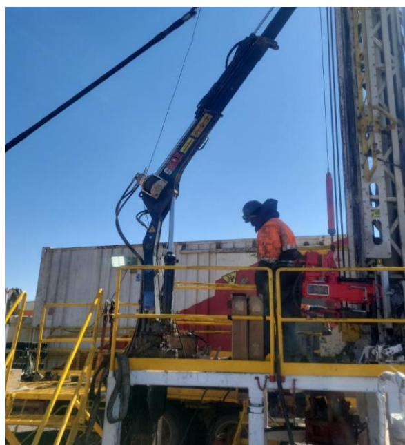
Workover rig at Nomgon-10
