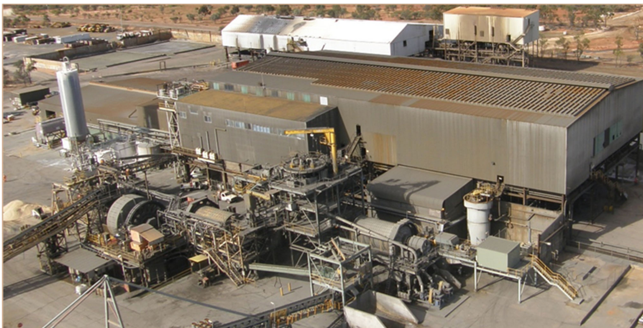
Figure 1: Endeavor Mine Processing Plant
