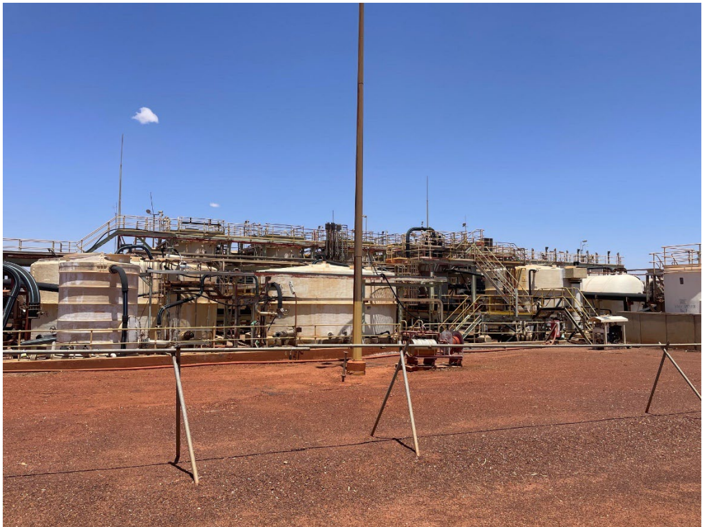
Figure 2-7: Solvent extraction plant
