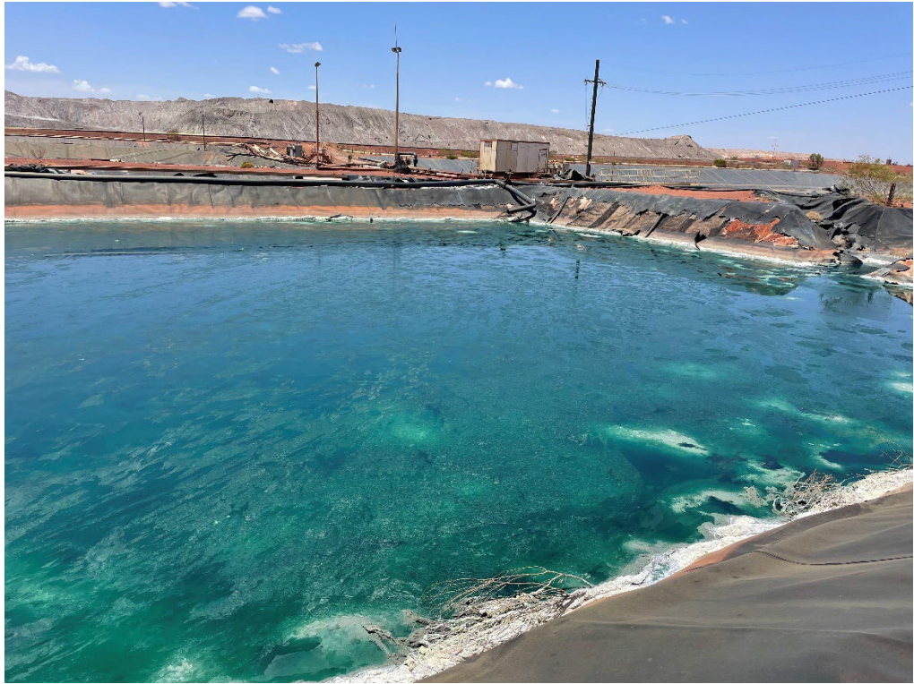
Figure 2-6: Pregnant leaching solution in pond
