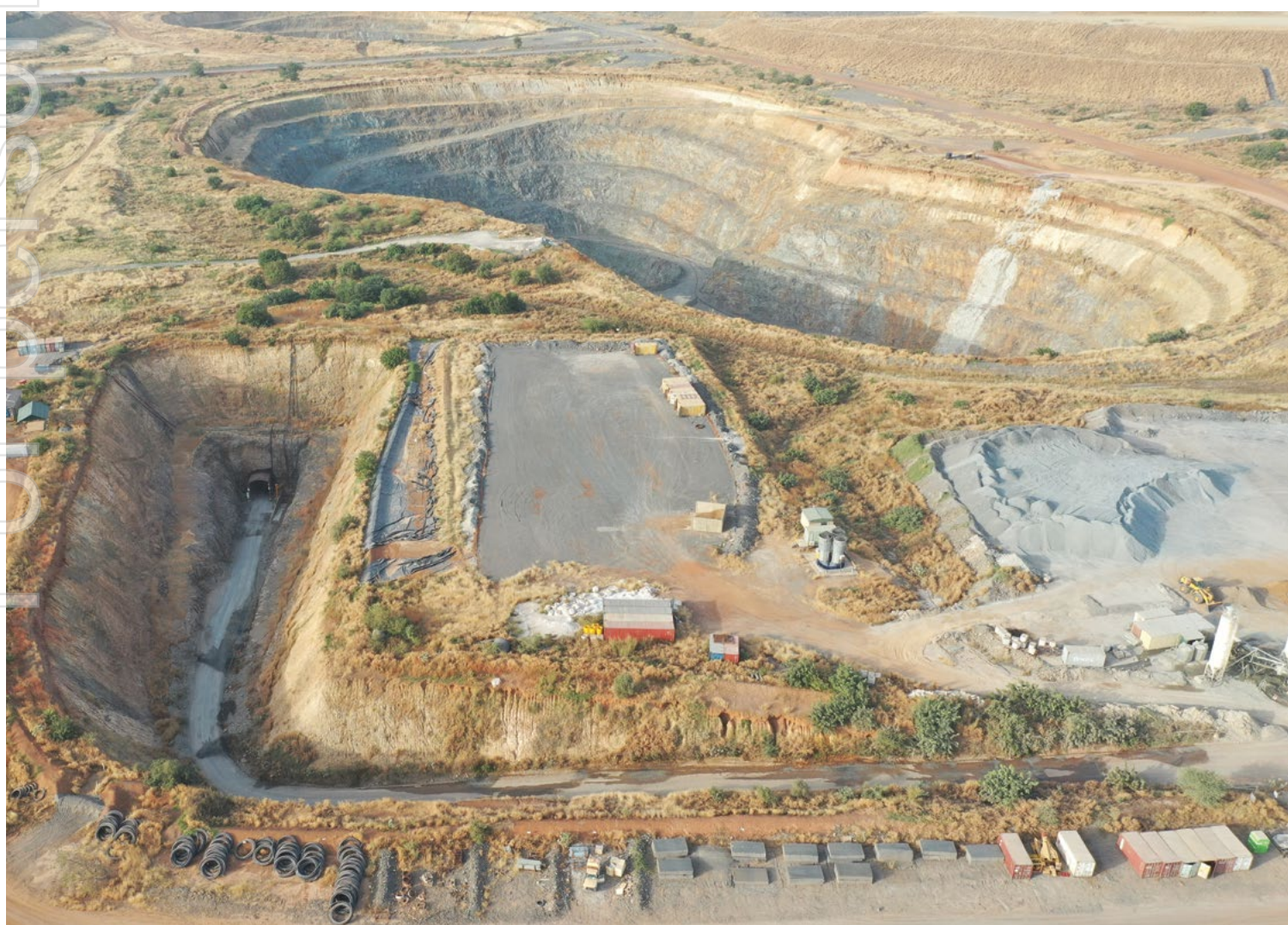
M1 Underground access portal
