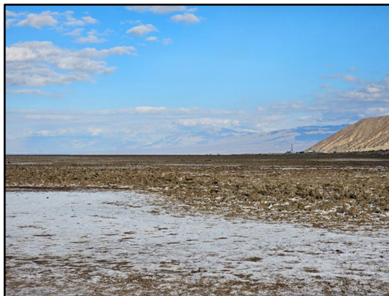
Figure 7: The drill rig on the first drill hole as seen from the second hole site at the Liberty Lithium Brine Project
