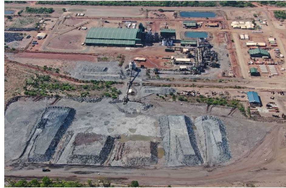
Process plant, product warehouse and ROM stockpiles
