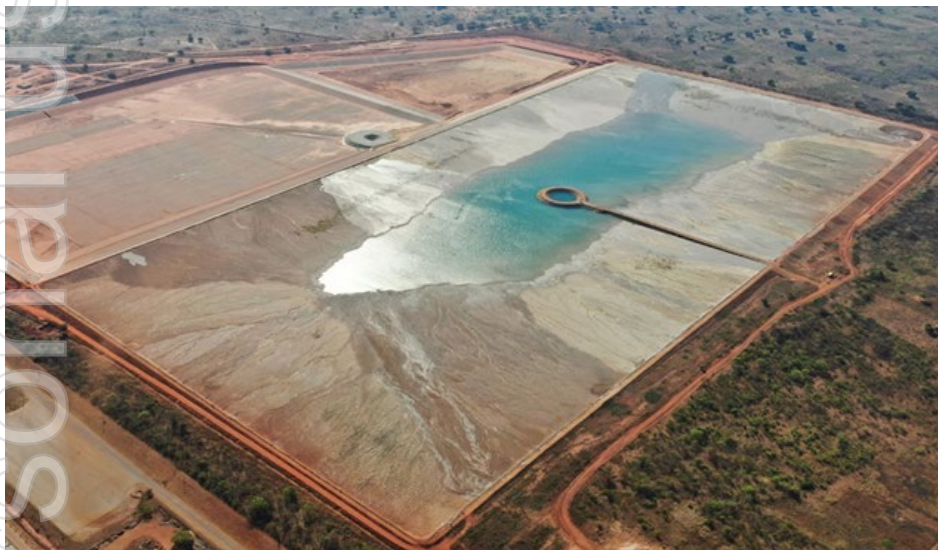
Tailings storage facility (cells 1 & 2)
