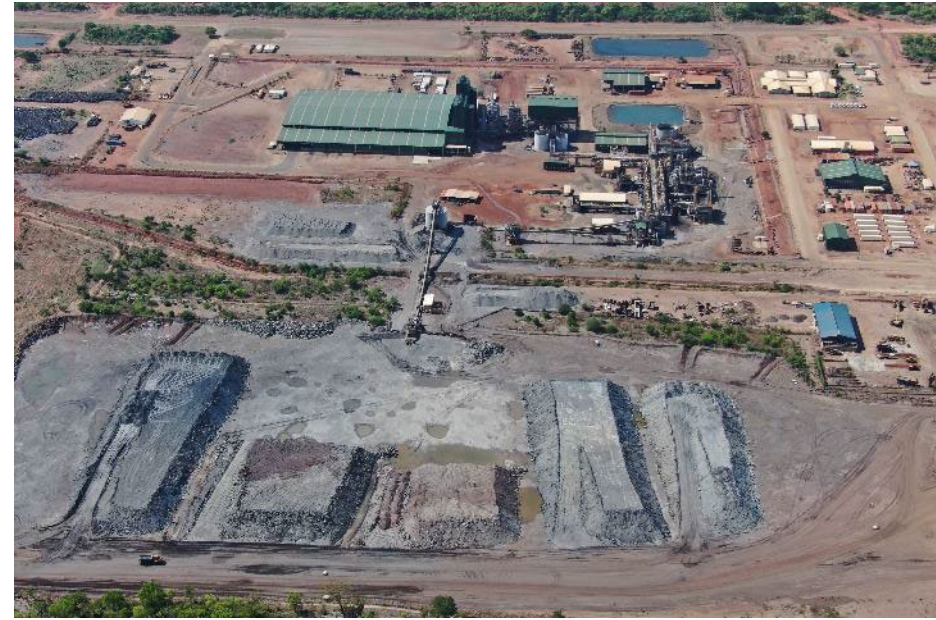
Process plant, product warehouse and ROM stockpiles
