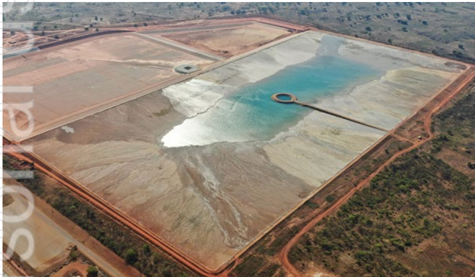
Tailings storage facility (cells 1 & 2)
