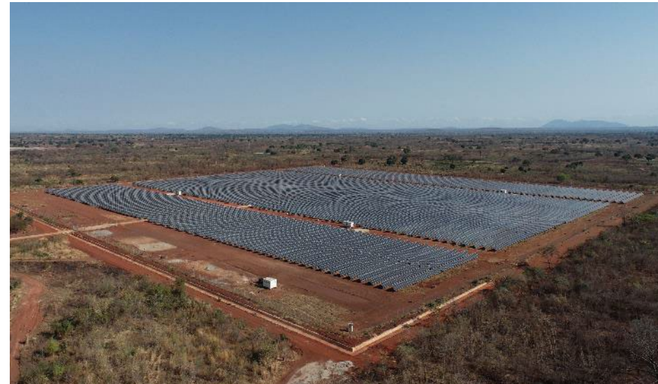
11.25 MWp solar photovoltaic array
