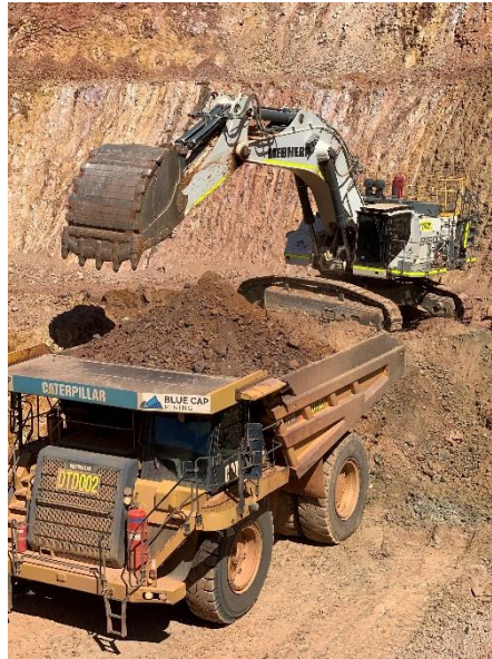
Figure 19 Typical excavator/truck combination
