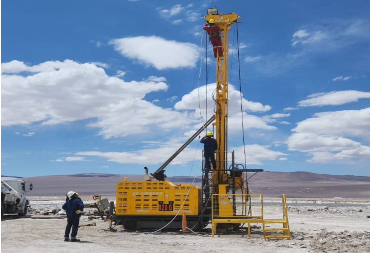
Figure 2 – DDH-1 drilling in progress
