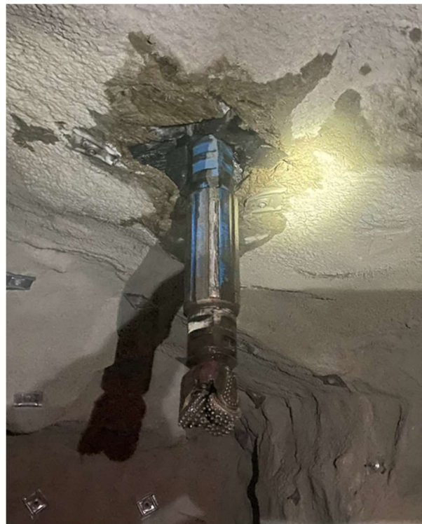
Figure 2: Pilot hole breakthrough
