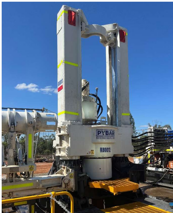
Figure 1: Pybar raisebore rig in place reaming
