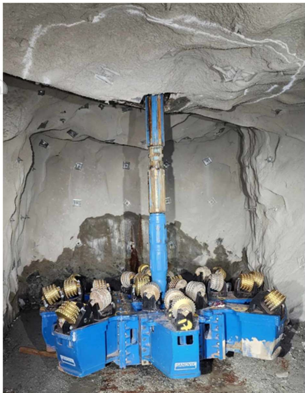
Figure 3: Reamer head being attached to rods
