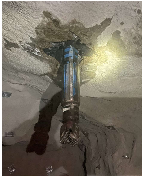
Figure 2: Pilot hole breakthrough
