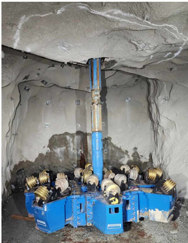
Figure 3: Reamer head being attached to rods
