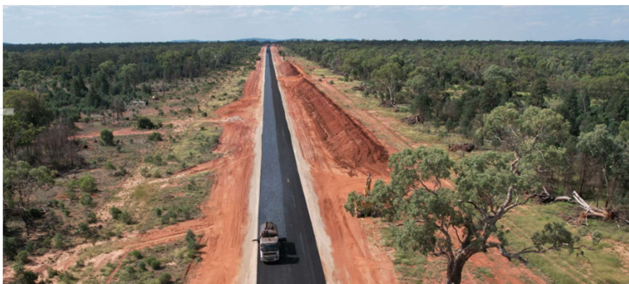
Figure 4: Road sealing works along the Burthong Road.
