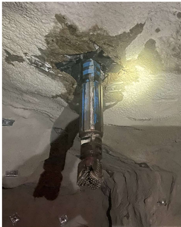
Figure 2: Pilot hole breakthrough
