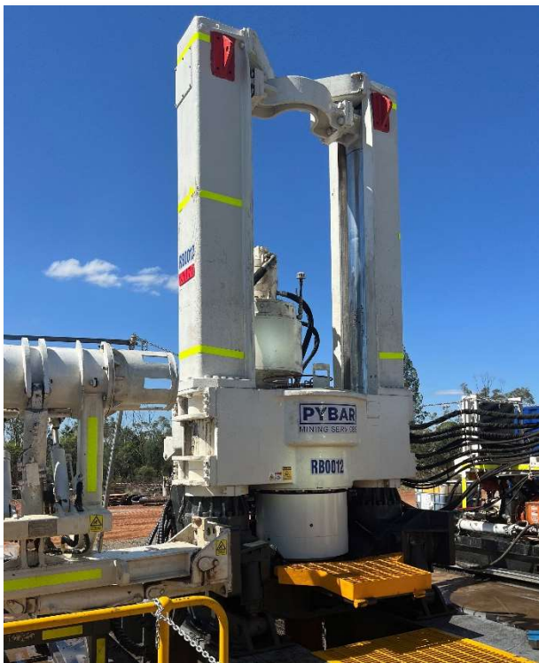
Figure 1: Pybar raisebore rig in place reaming
