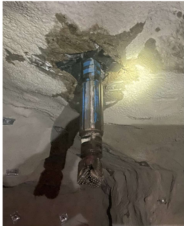
Figure 2: Pilot hole breakthrough
