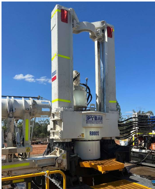
Figure 1: Pybar raisebore rig in place reaming
