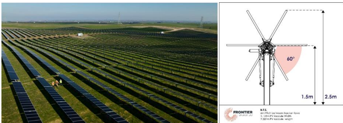
Figure 11: Typical solar farm arrangement with tracker
