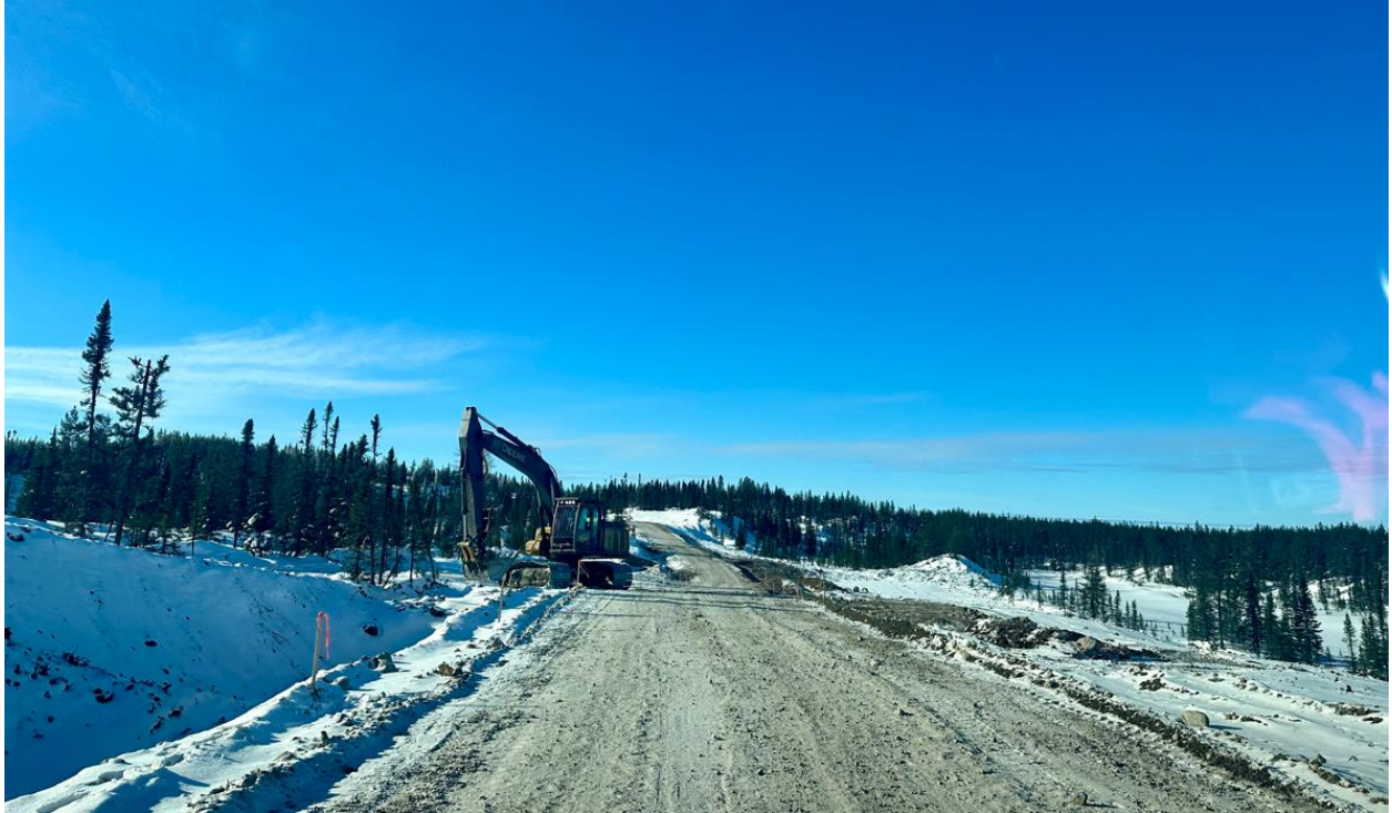
Figure 5: Portion of all-season road, constructed by the Company, extending south from Shaakichiuwaan Camp, at KM-270 of the Trans-Taiga Road, to the CV5 Spodumene Pegmatite.
