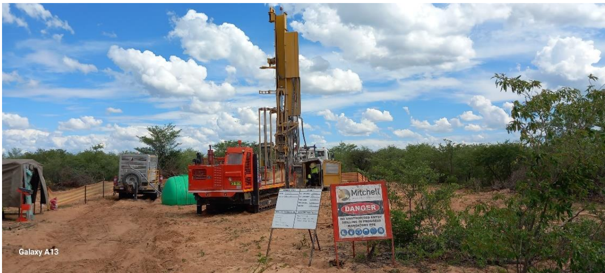
Hydrogeological drilling, NCP Botswana
