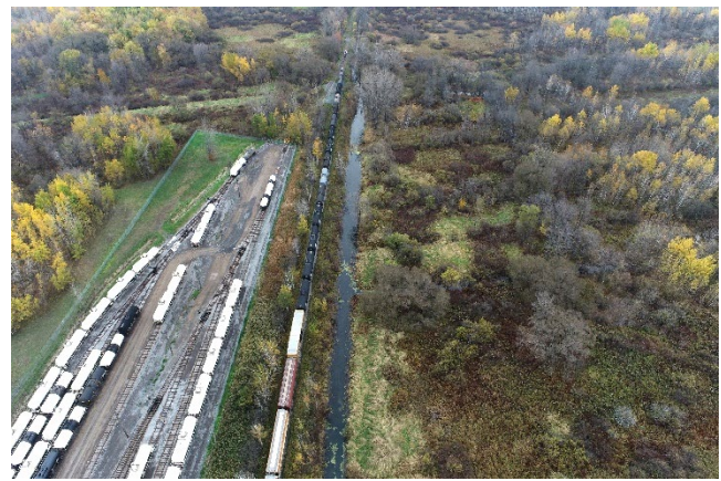
Figure 4: North side of Lot 22 at Bécancour, Québec proximal to rail infrastructure.
