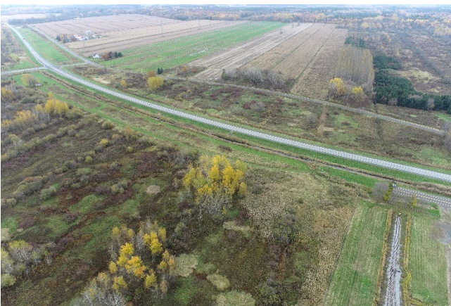
Figure 3: South side of Lot 22 at Bécancour, Québec proximal to highway access.
