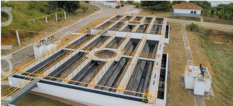
Sewage treatment plant, Colatina
