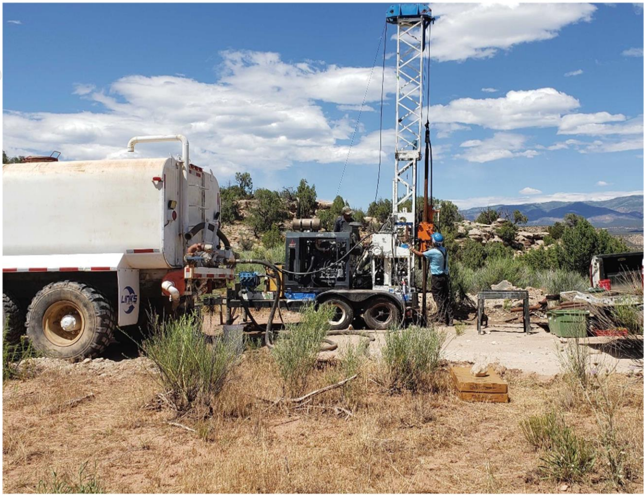
Figure 2 – Drill rig on site – REX Project
