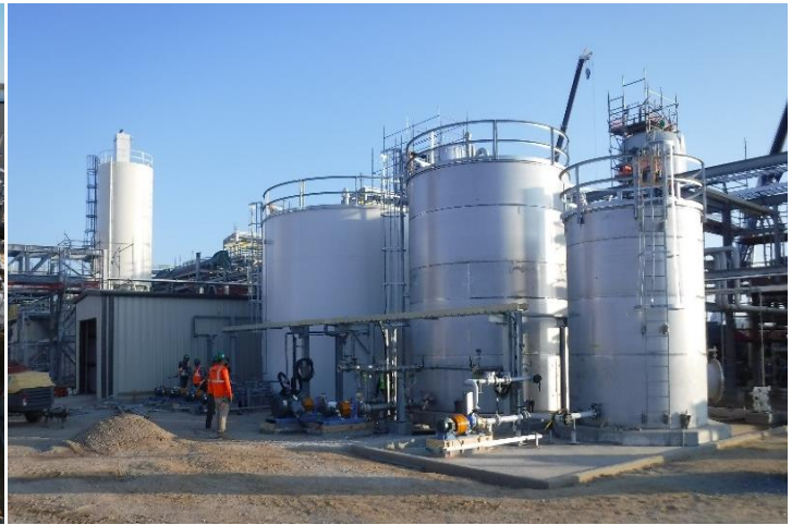
Figure 4: Vidalia 11.25ktpa AAM facility air compressors (left); water and neutralisation discharge tanks (right).
