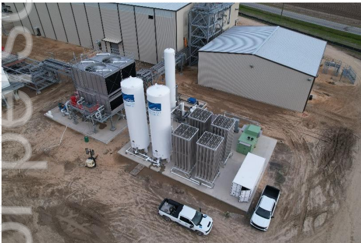
Figure 5: Vidalia 11.25ktpa AAM facility nitrogen plant (left); power distribution centre (right).
