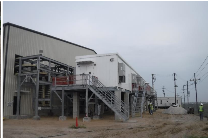
Figure 5: Vidalia 11.25ktpa AAM facility nitrogen plant (left); power distribution centre (right).
