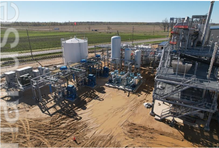
Figure 4: Vidalia 11.25ktpa AAM facility air compressors (left); water and neutralisation discharge tanks (right).
