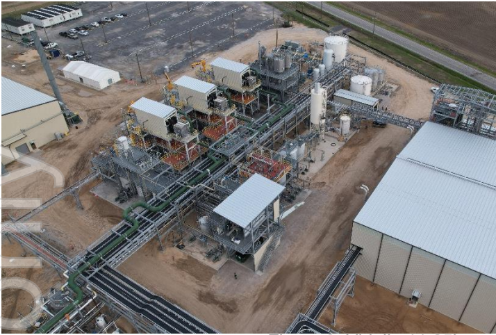
Figure 3: Vidalia 11.25ktpa AAM facility purification area.
